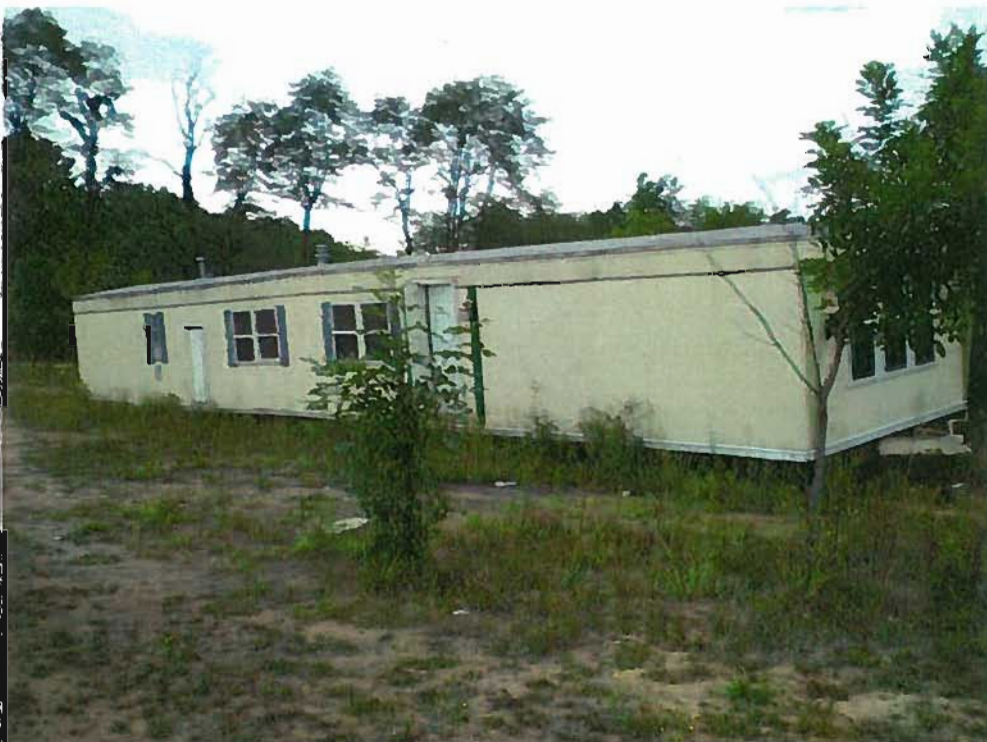
Date: September 14, 2011 Time: 12:17 PM Direction: Northeast Photo by: W Zierath Exposure #: 016 Comments: An uninhabited mobile home in the north part of the site.
